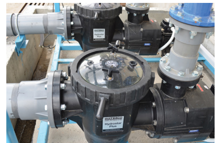
Compared to steel pumps, Hydrostar Plus is made from high-quality engineered plastic that is chemical resistant and durable in all weather.
